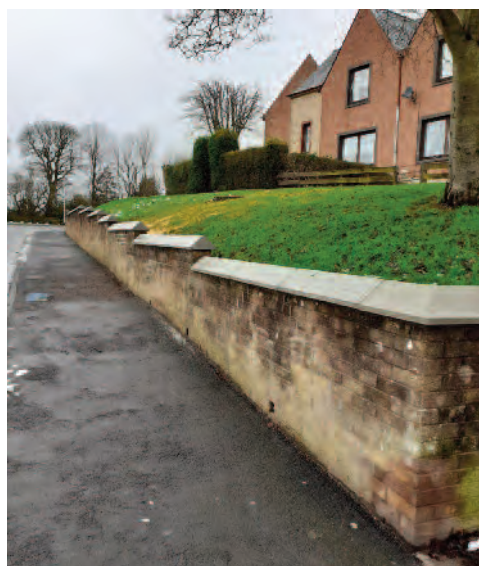
Improvements to wall, Burnfoot
