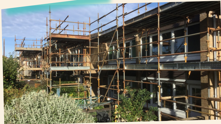
Programme of external works at Tweed Court, Kelso currently underway
